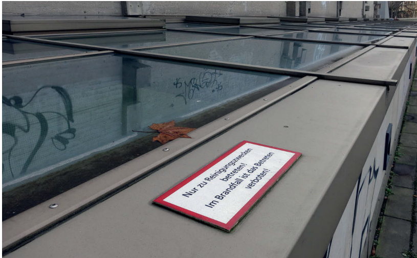
Figure 2.11.: Accessible glazing with sign: "Enter for cleaning purposes only! Do not enter in case of fire!". Schneider Glasbau [110].
