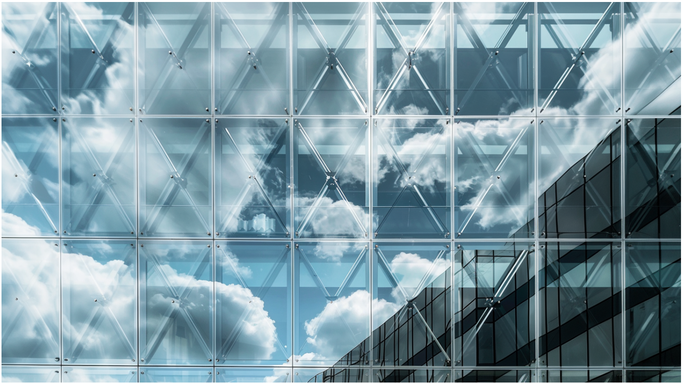
Figure 6.5.: Visualization of a fully glass facade, which was stiffened by local bending or AM imprint in cross shape [93].
