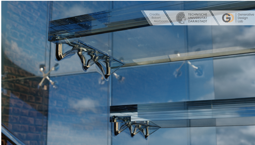
Figure 1.25.: Connection of glass stair treads to flat glass using AM.
