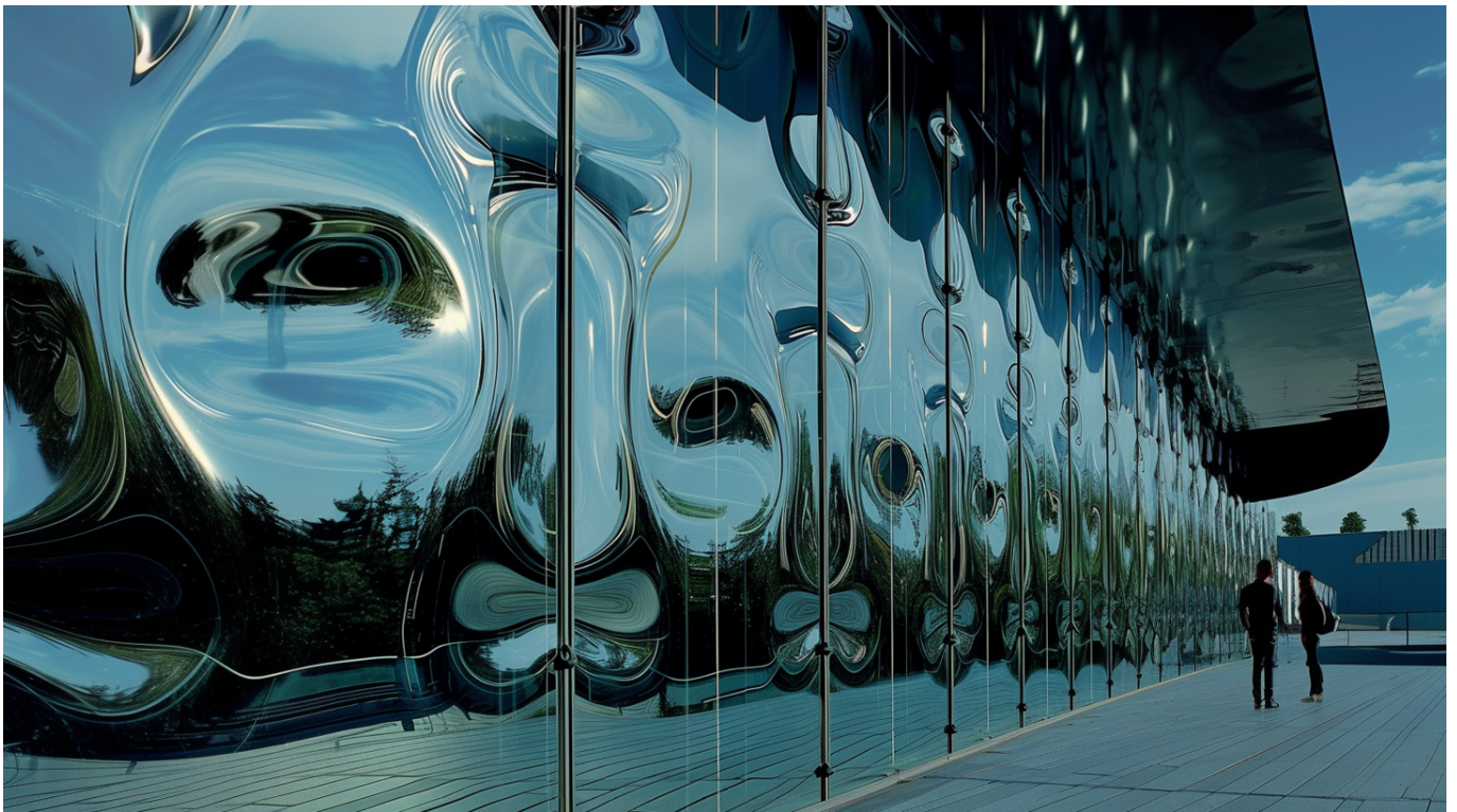
Figure 6.4.: Visualization of a locally curved glass to increase the moment of inertia [93].
