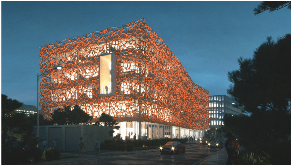
Figure 1.12.: 3D-printed facade in Regensburg, Germany produced and designed by additive tectonics GmbH [68].
