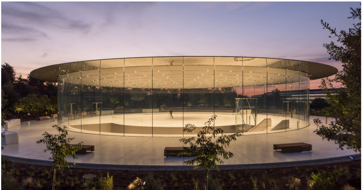
Figure 1.18.: Glass as a structural element in the Steve Jobs Theater. Photo by Foster + Partners [57].
