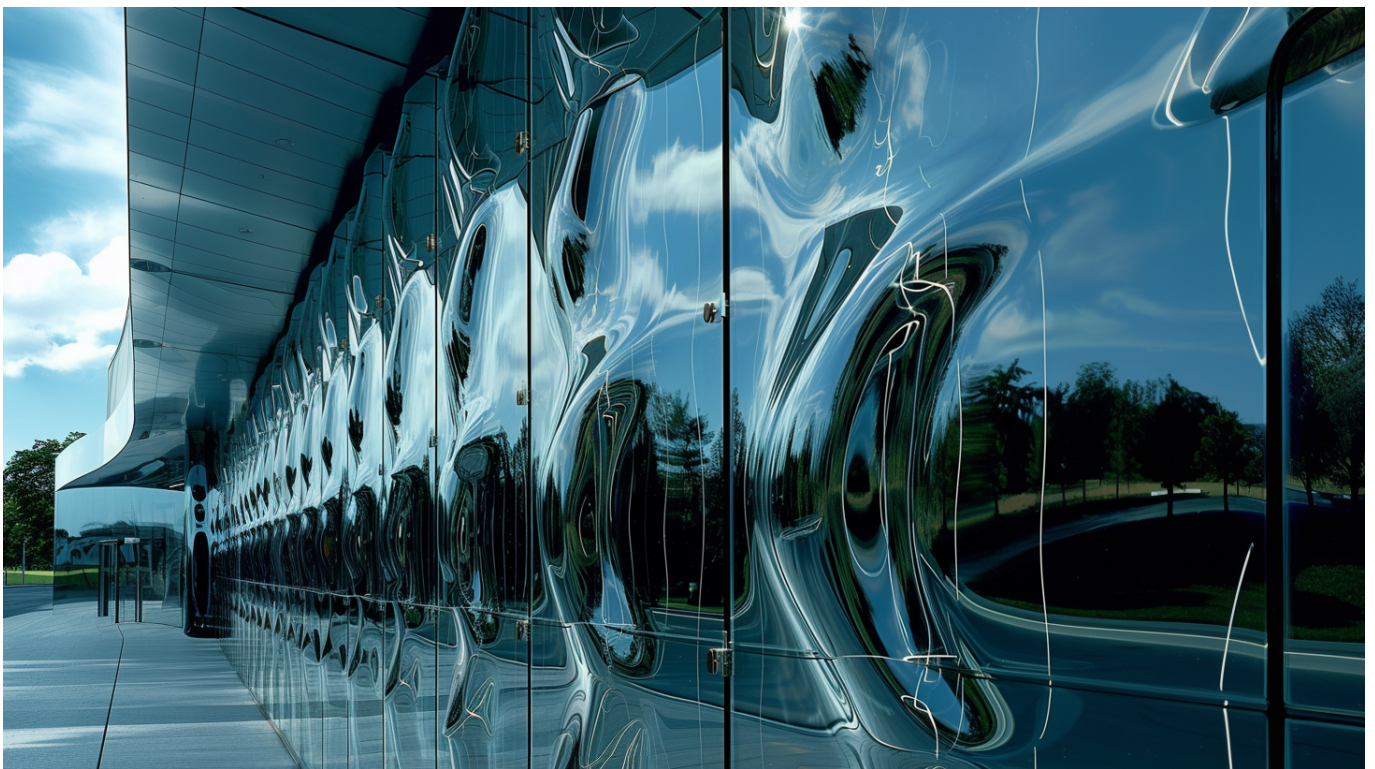
Figure 6.8.: Visualization of a locally curved glass to increase the moment of inertia [93].
