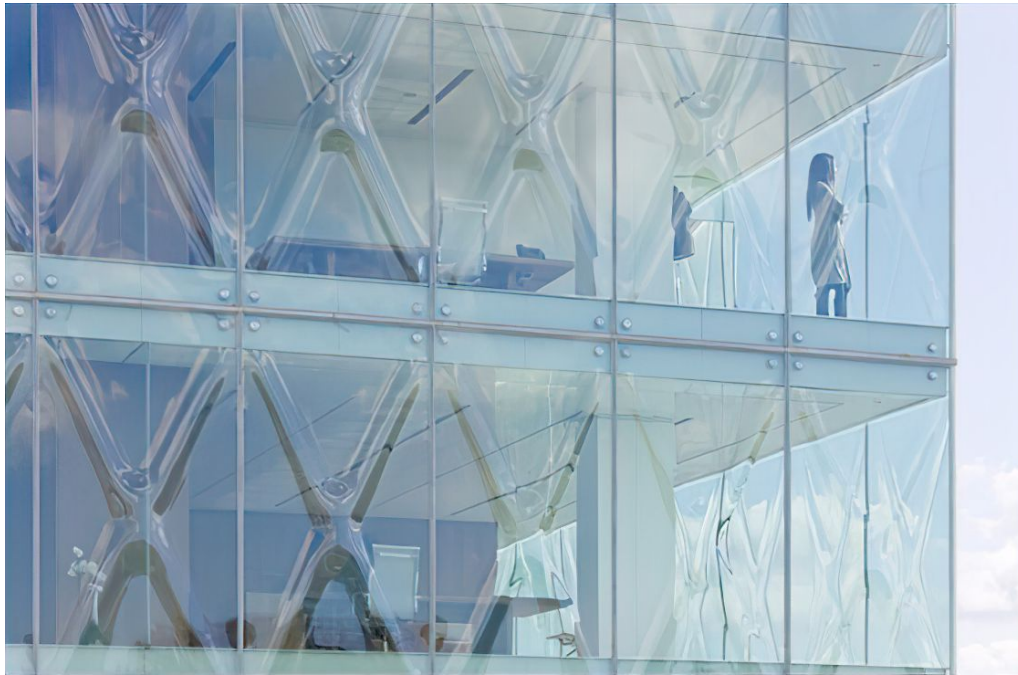
Figure 1.27.: VAKKO® headquarter in Istanbul, Turkey. The facade is fitted with glass panels that have gained stiffness through a deep-drawing process [123].
