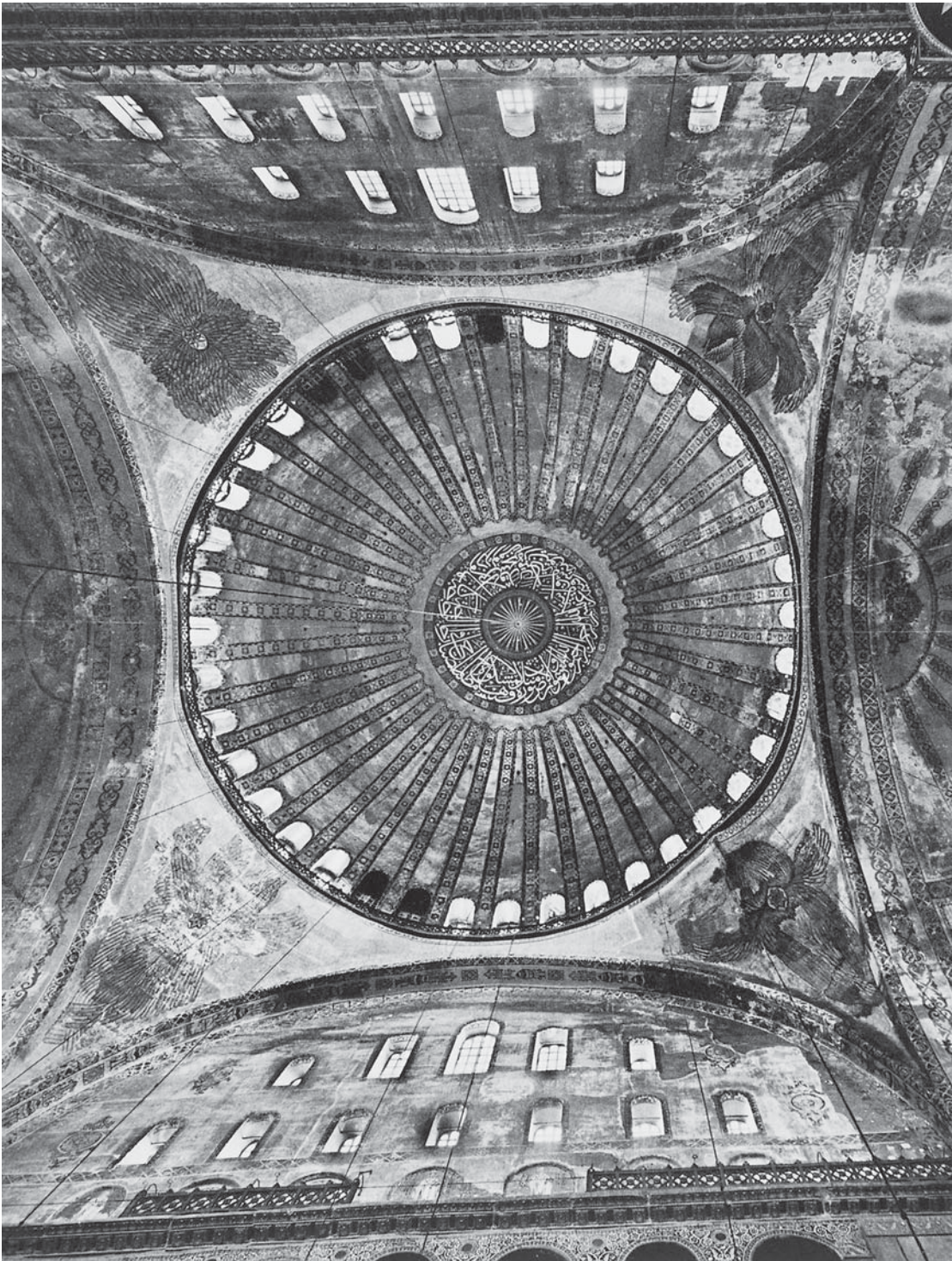
Figure 1: Hagia Sophia in Istanbul. View into the dome and the pendentives; (Kähler 1967, pl. 27)
