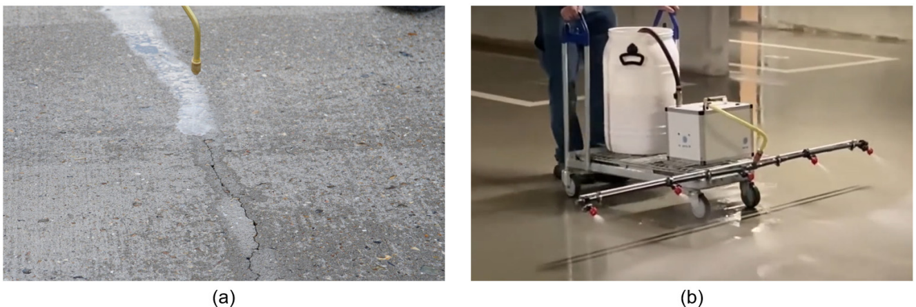
Figure 4-1: Two application methods of Basilisk ER7: (a) jet spray and (b) complete surface treatment (Basilisk, 2021g)
