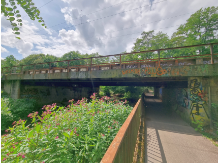
(a) Side view of the bridge
