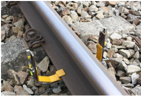
(a) installed sensor (photo: Hagen Berthold)
