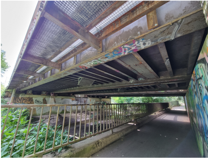
(c) View of the load-bearing structure from below
