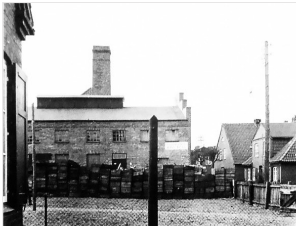
Fig. 2.21 Fish-factory-converted church in Schlutup Source: Emil Steffann (1899-1968): Werk, Theorie, Wirkung (Haus, 1999)
