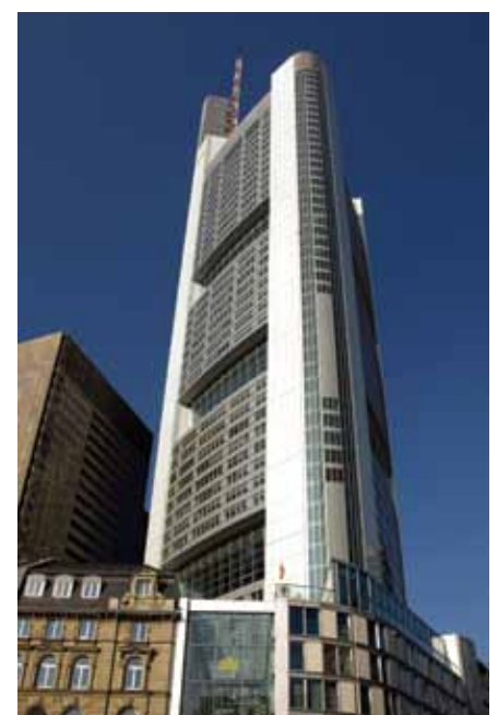
Figure 4. Commerzbank Tower, Frankfurt. © Marshall Gerometta
