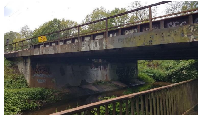
Figure 1 Examined single-span steel trough bridge.
