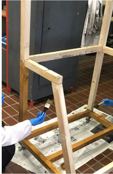
Figure 4.4: Application of the fire-retardant paint on wooden structures.
