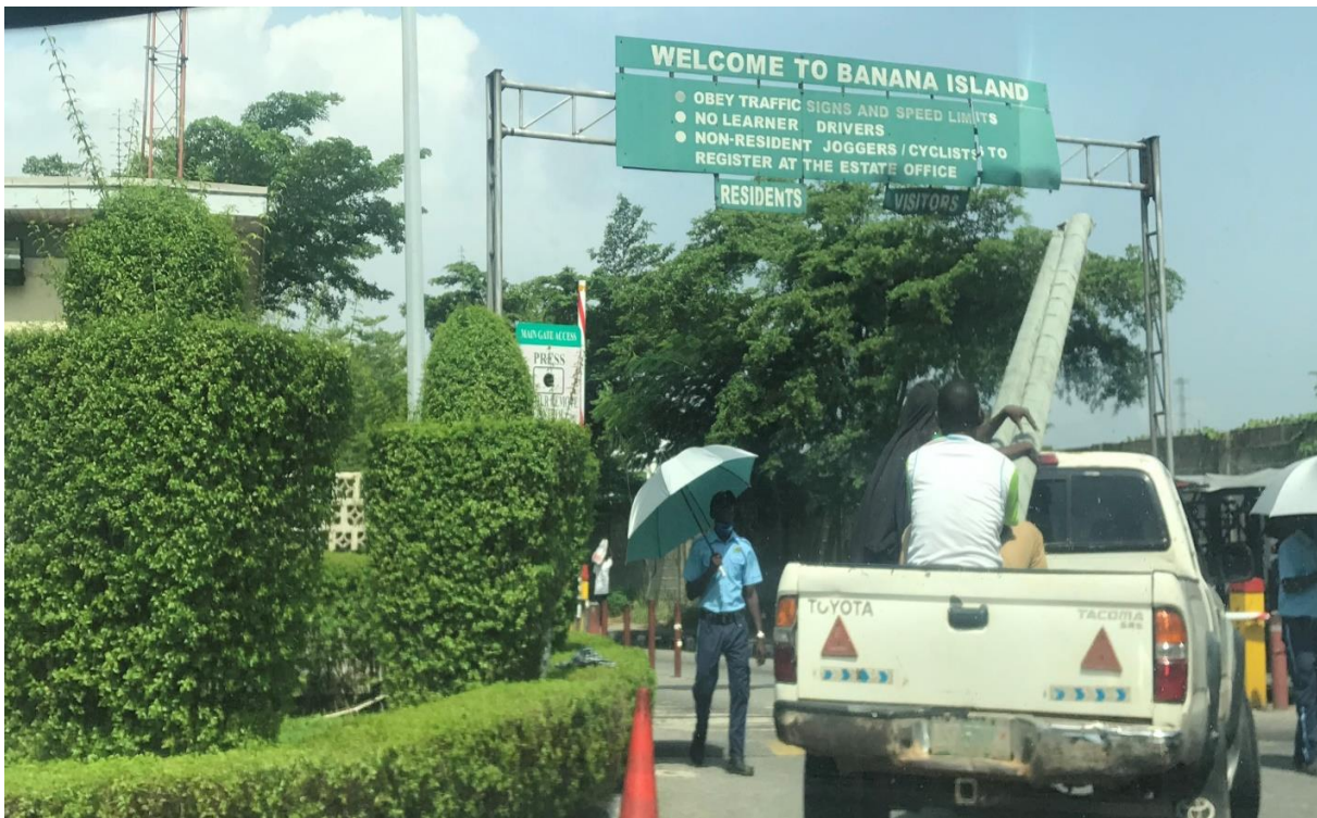
Plate 5.1: Vehicular check/control at Banana Island's main entrance. (Source: author, 2020)
