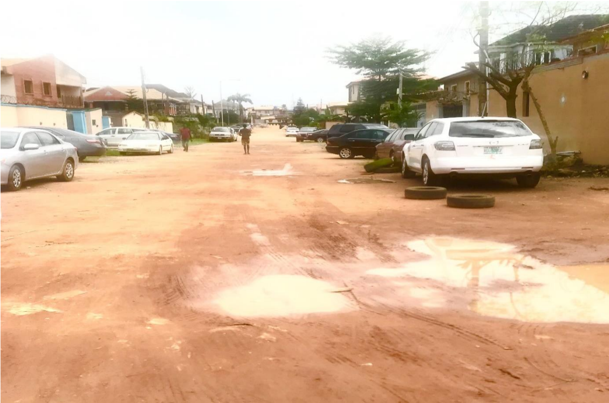
Plate 5.6: An untarred street in Omole Phase II (Source: Author, September 2020)
