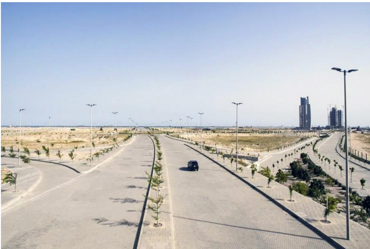
Plate 6.9: Image of the 8-lane, 1.5km-long Eko Boulevard that runs from the Ocean Front into the Ahmadu Bello way. It is Nigeria's first 8-lane city road (Source: media on www.ekoatlantic.com ).
