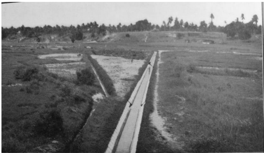
Figure 3.10: Gerezani Creek Concrete-Lined Drainage, 1936 Source: R Mackay, Second Report of the Malaria Unit, Dar es Salaam, 1938.
