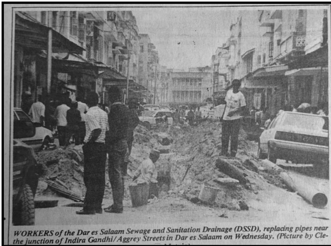
Figure 5.9: Major Repairs of Combined Drainage in 1992
