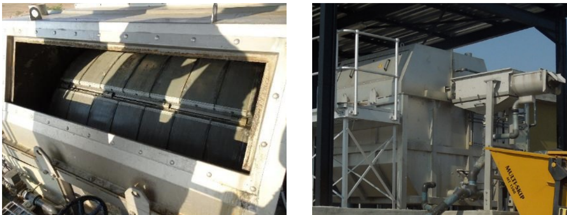
Figure 2.3: Micro sieve with sieving drum (left) and screening discharge (right)
