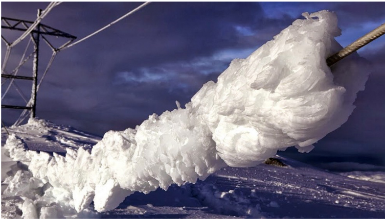
Figure 1.4: Transmission line at Ålvikfjellet, Norway collapsed due to icing. Photo reprinted from Engdahl et al. (2020).
