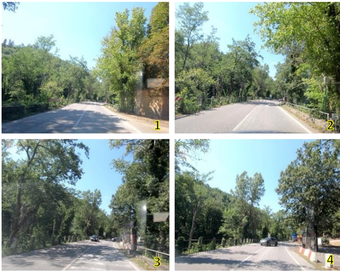
Figure 3.55 – Sequence of photos approaching an “invisible” intersection, starting 70 m ahead of the intersection. The last photo is about 25 m before the intersection (photo by Andrea Paliotto)
