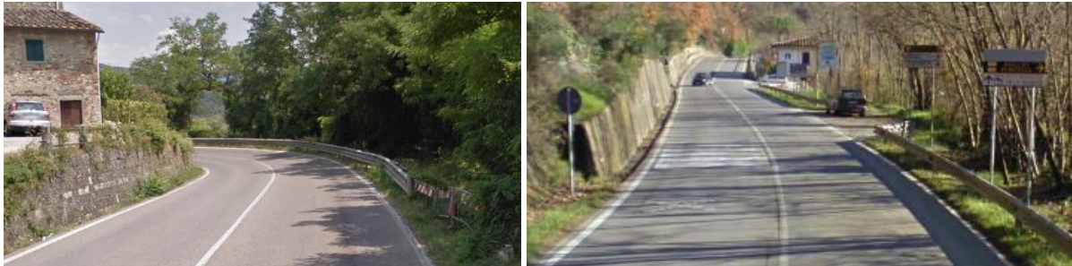
Figure 5.3 – Photos of SR206: on the left km 282.100 northbound, on the right km 288.400 southbound.
