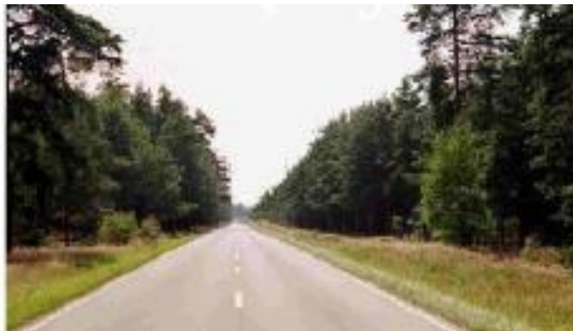
Figure 3.56 –Optical orientation to the horizon: distant focus and monotony decreased workload and cause subconscious acceleration. Furthermore, the road is not in the center of the space between the trees, and this can cause an unconscious shifting in the lane, from Birth (Birth, 2009)
