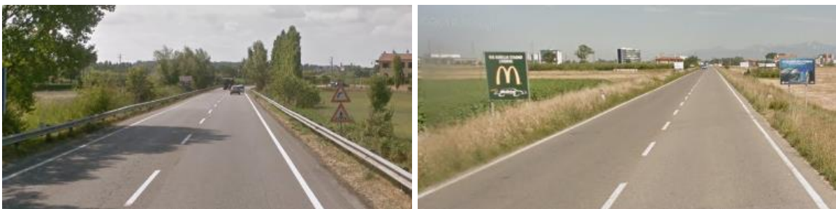
Figure 5.4 – Photos of SR206: on the left km 33.700 southbound, on the right km 39.200 northbound.
