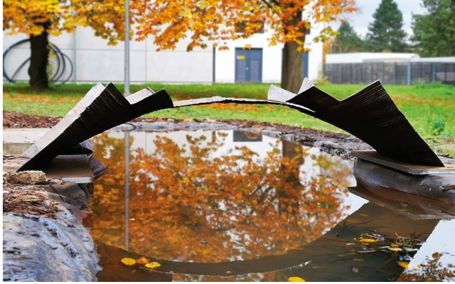
Fig. 22 The bridge after closure of the span
